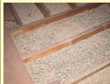
A close up of Vermiculite in an attic.
